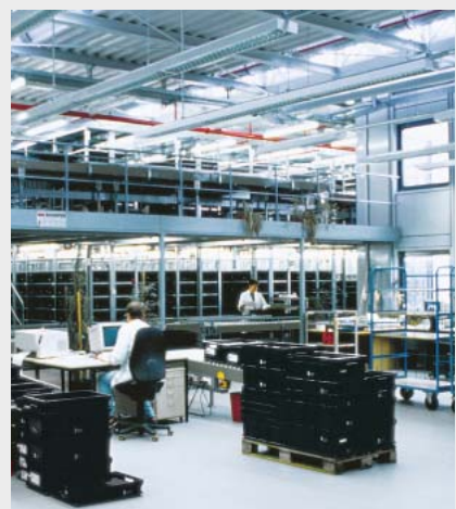
Precision work is made easier by neutral white light colour 940 with optimum colour rendering.
